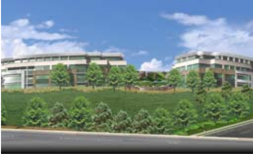
Gateway at Torrey Hills
